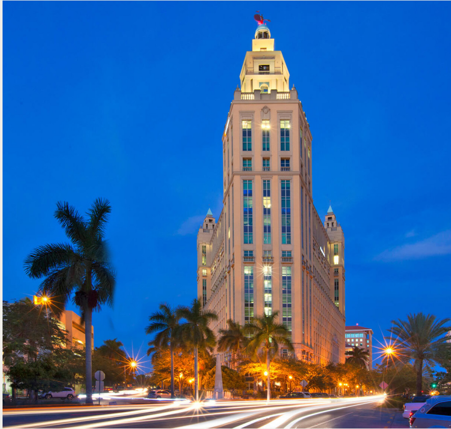
Alhambra Towers, Coral Gables, FL
